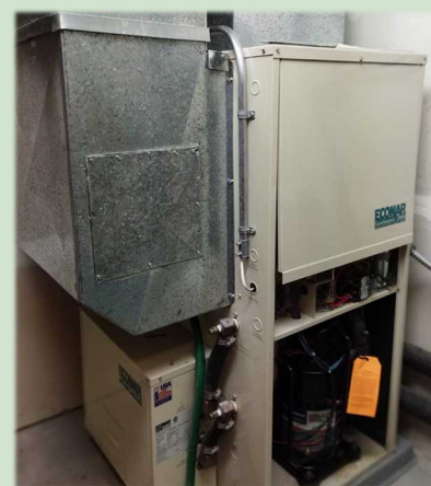
One of seven heat pumps that need replacing.
